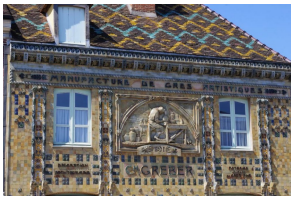
Exterior view of a building facade
