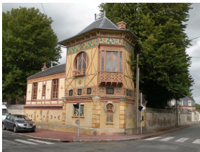
Exterior view of a building facade
