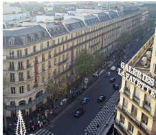
Boulevard Haussmann, lined with typical Haussmann buildings.
